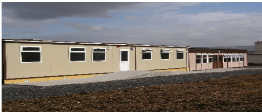
A view Of Our New Classrooms at Coola
